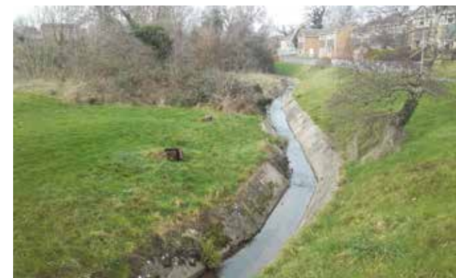
Work involved removing this concrete watercourse
