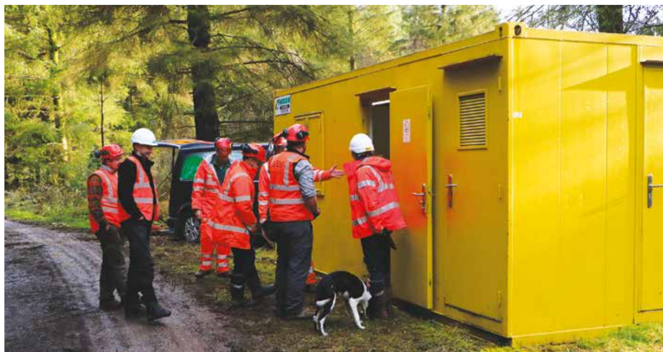
Typical welfare unit on site
