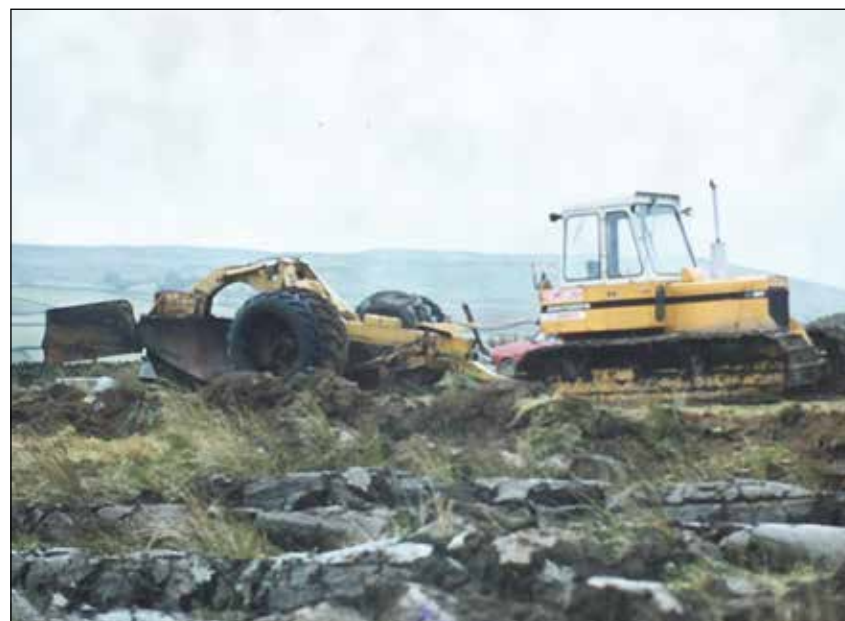
The humpy plough starting the drainage works.
